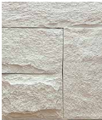
5 Seam Filling Color Repair
